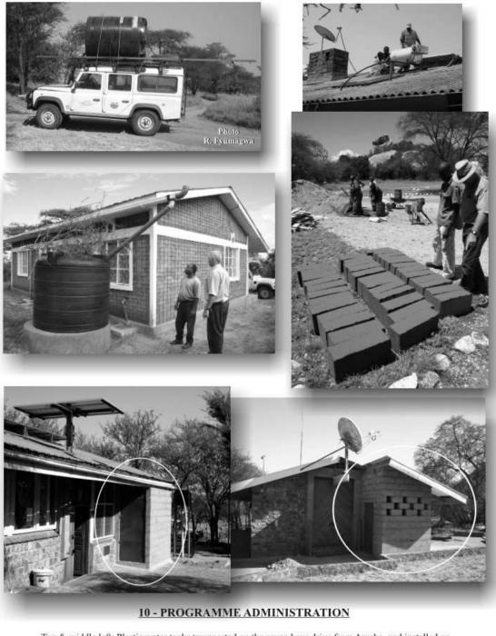
Top & middle left: Plastic water tanks transported on the seven hour drive from Arusha, and installed on staff housing. Top right: Solar water heater on roof at staff housing Middle right and below: Battery and generator rooms for power system upgrade at the laboratory built with concrete blocks made on site.
